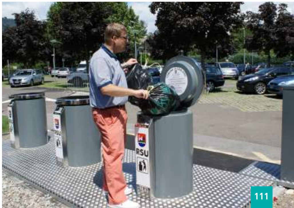
The throw-in can only be opened using an access card.
