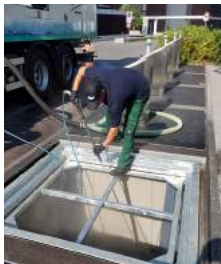
Interior cleaning of concrete with high-pressure cleaner.
