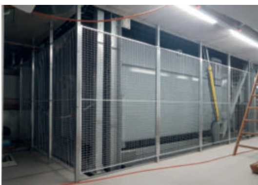
Lift system with fencing on all sides.
