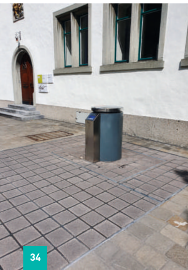
Left: Caslano type throw-in column with access system integrated with the disposal hatch. Platform with paved surface.
