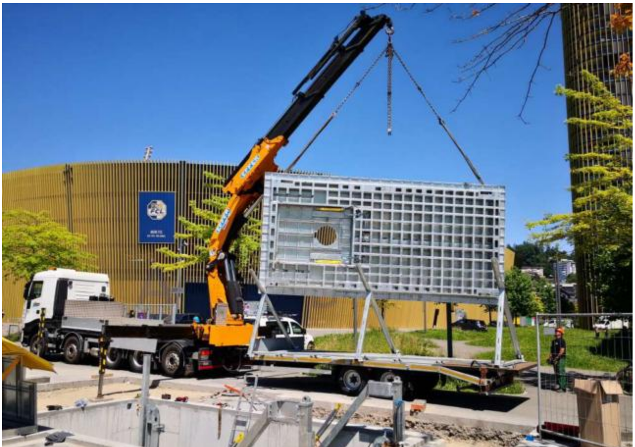
Transport of a platform and associated installation work.
