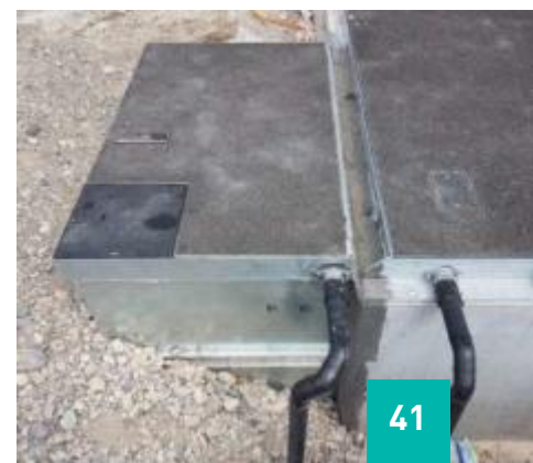
Drainage pipes, technician shaft and platform
