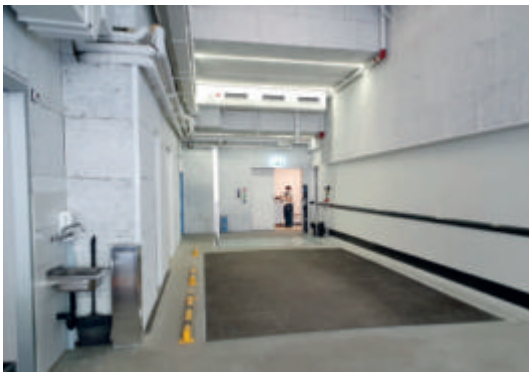
The lift platform can take the weight of trucks up to 40 tons.
