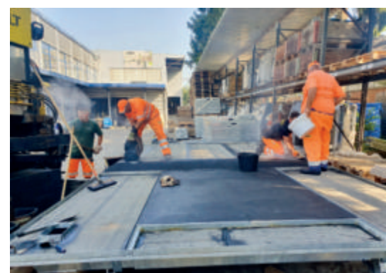
Laying mastic asphalt
