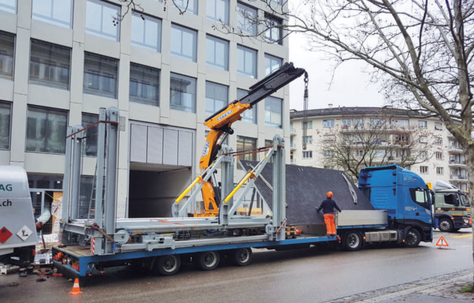
Left: Assembly work of a lift system.
