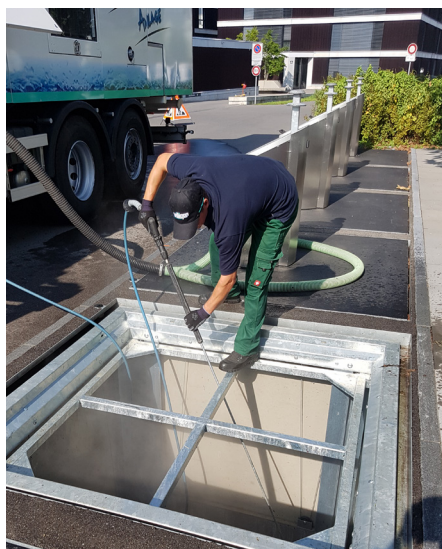
Interior cleaning of concrete with high-pressure cleaner.
