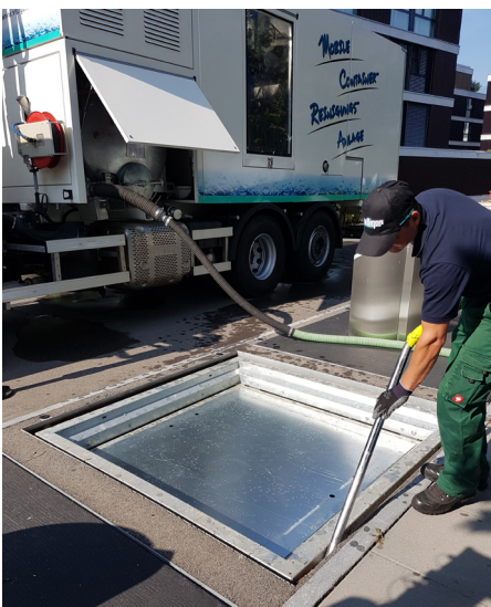
Suctioning residual dirt such as water and leaves.
