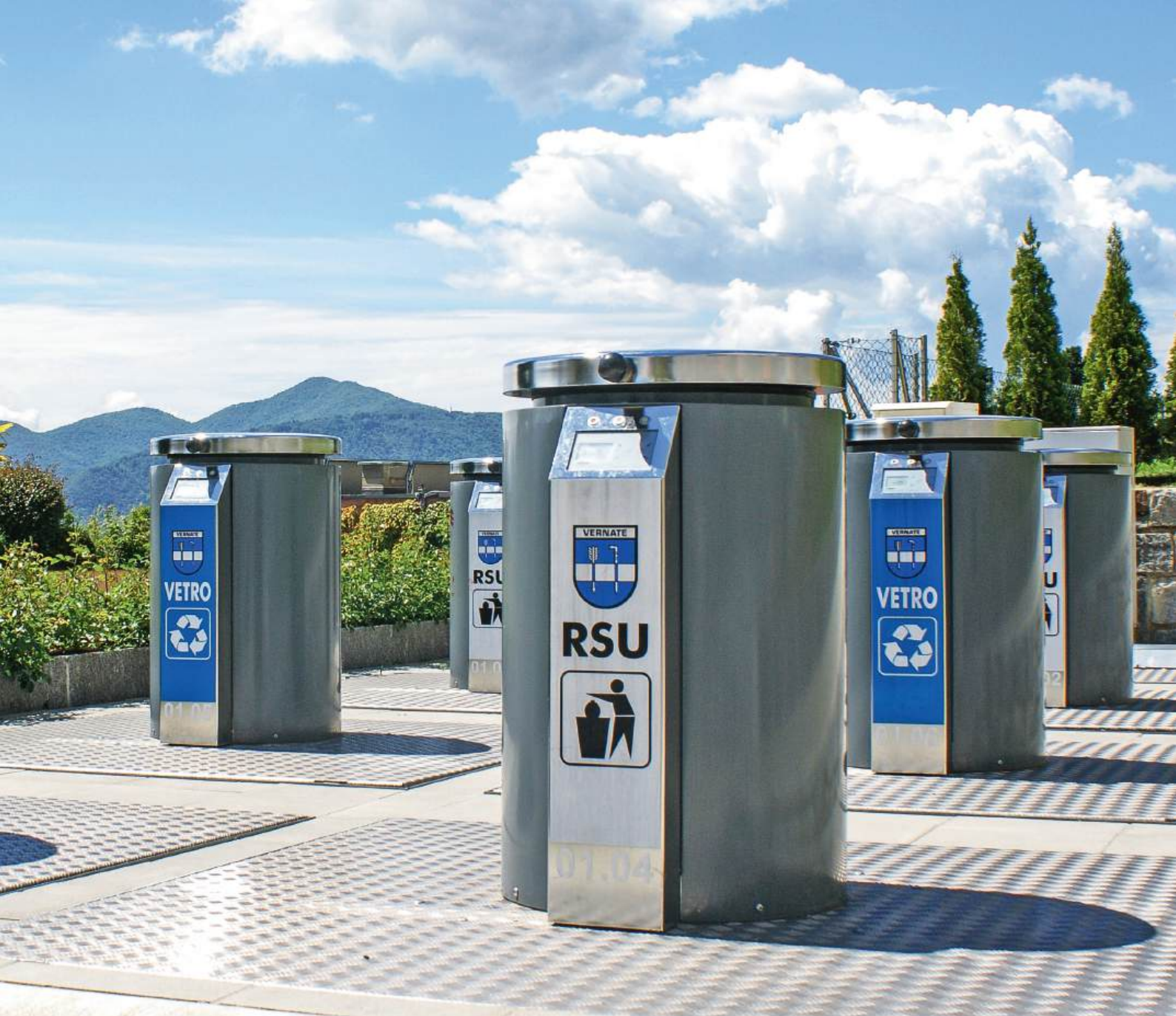
Collection point with Caslano throw-in columns and electronic access with weighing.
