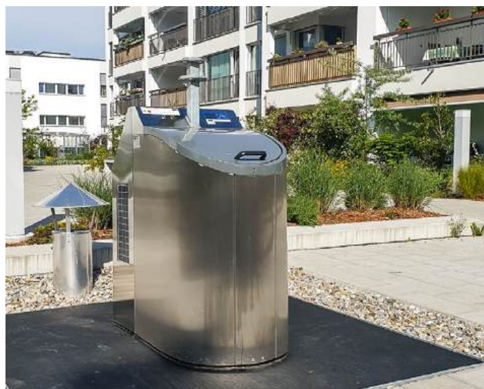
Underground system with Vilaro throw-in column with electronic access/weighing and solar power supply.
