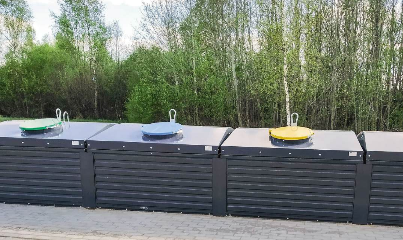
Semi-sub with trapezoidal sheet metal cladding.
