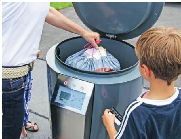
After closing the lid, the weight of the waste is recorded.
