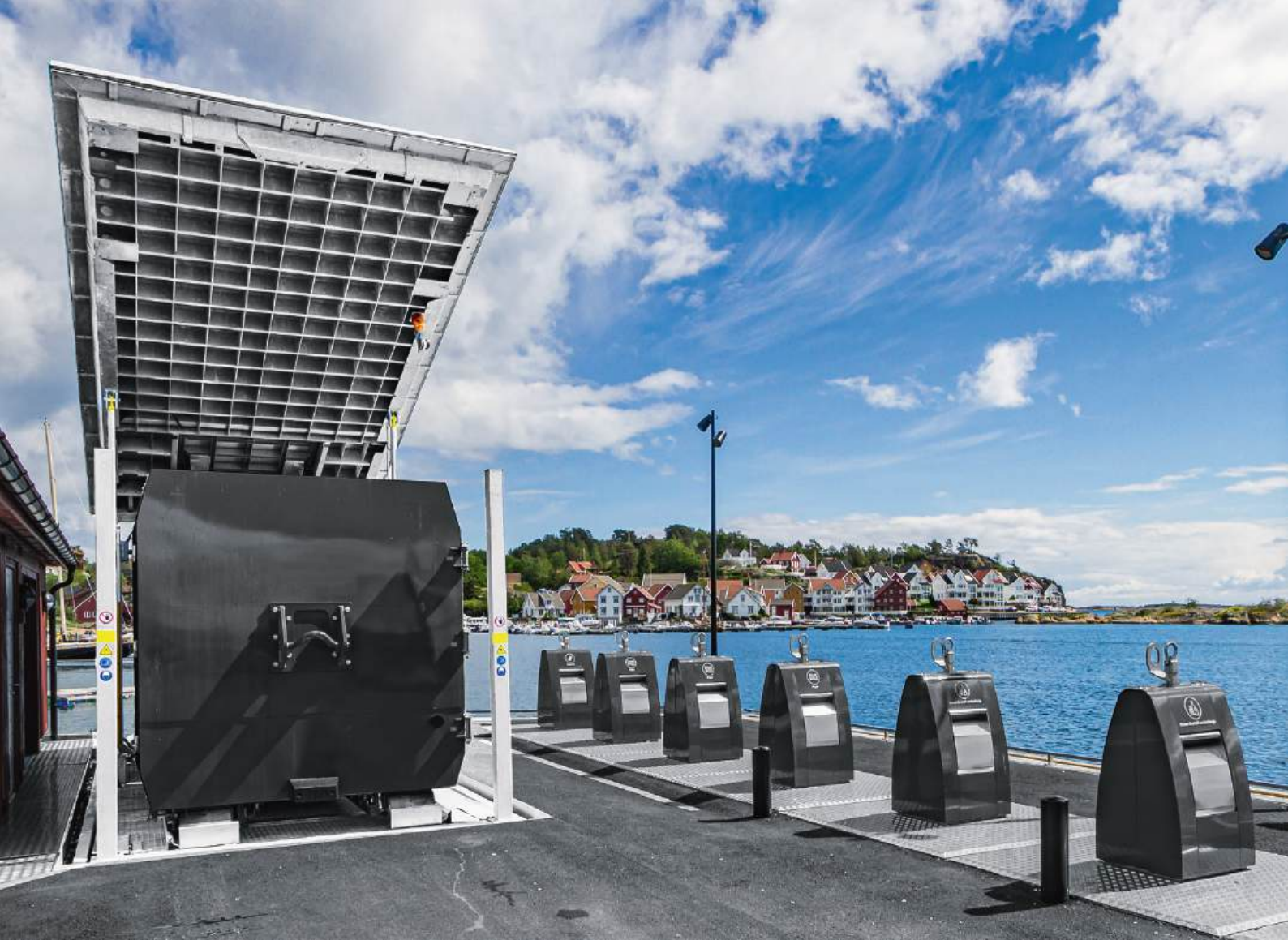
Up to 20 m 3 of compacted waste is collected in the underground press container on the coast of Norway. The disposal costs are thus significantly reduced.
